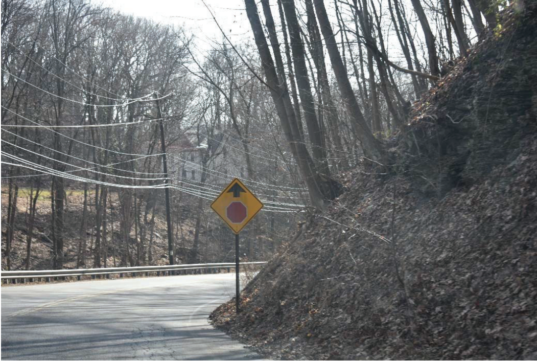
Sight distance in horizontal curve approaching stop sign at Beaver Street
