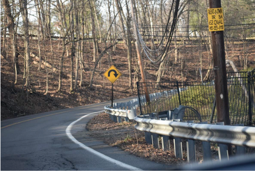
"Hairpin Curve" sign (W1-11) in the northbound direction. A second sign is installed southbound.
