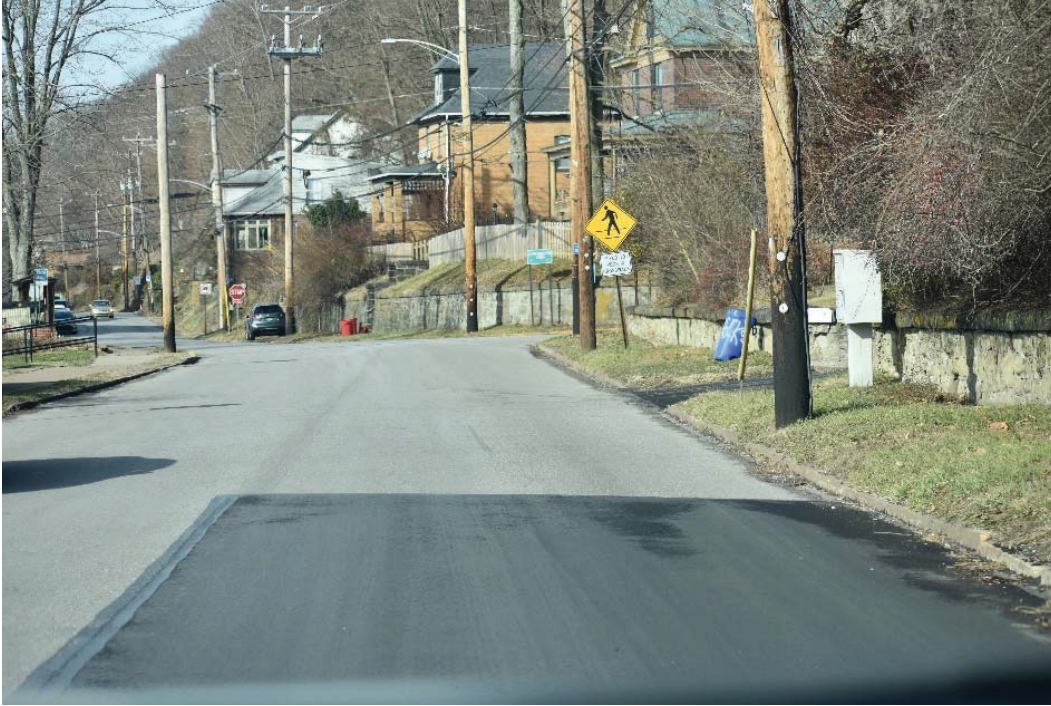
Photo shows skew in Beaver Street at its intersection with Camp Meeting Road. It also shows the lack of pavement markings.
