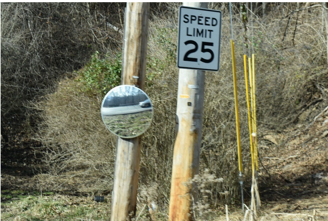
Mirror at a driveway along Camp Meeting Road due to poor sight distance
