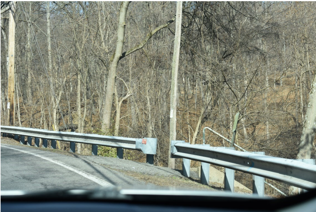
Earth around guide rail posts is eroding away from the posts in the background of the photo.
