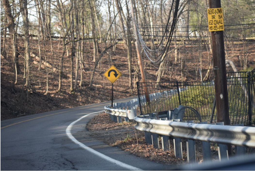
"Hairpin Curve" sign (W1-11) in the northbound direction. A second sign is installed southbound.
