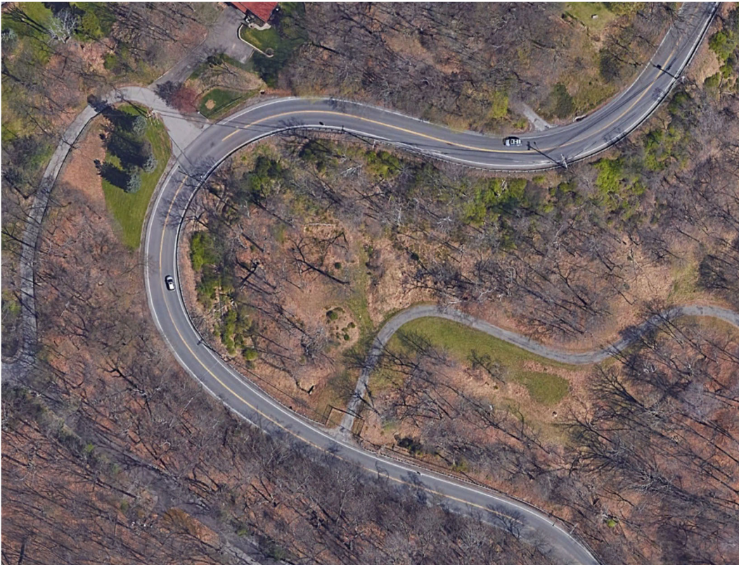
Curve with “Hairpin Curve” (W1-11) sign installed
