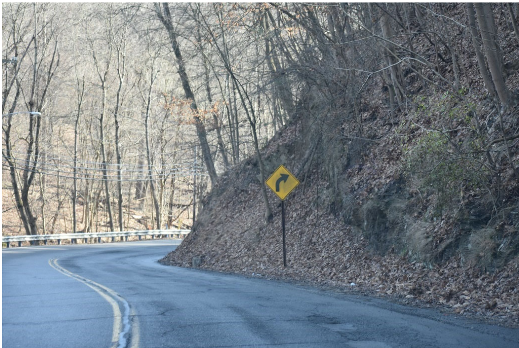
Sight distance in horizontal curve approximately 1200-ft from Beaver Street
